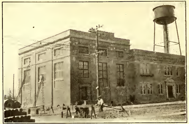
MILWAUKEE CARHOUSE AND STATION—SUBSTATION AND TRAINMEN'S BUILDING
